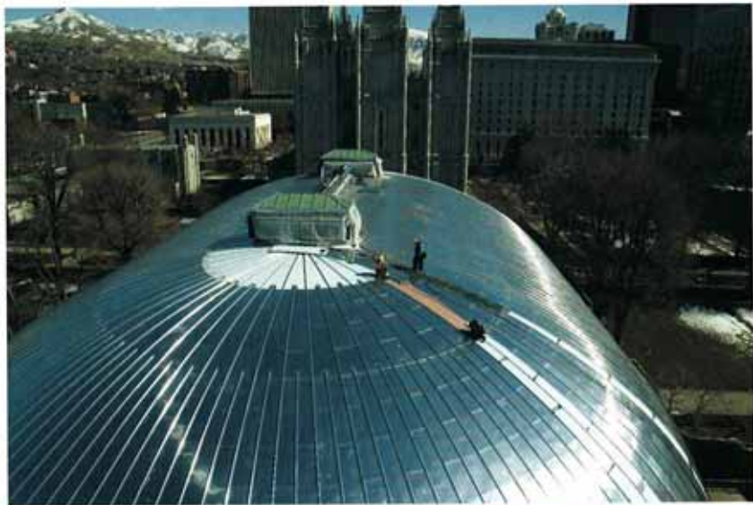
Top: The attic space beneath the tabernacle's spectacular dome now houses two Christie Digital Roadster HD12K HD DLP projectors.
